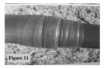
Next wrap each joint on the fiberglass poles with the all weather electrical tape, see **Figure 9**. Each joint should have at least the full width of the tape on both sides of the joint. Use common sense on the amount of tape or you will not have enough of the silicon tape used later to cover the electrical tape.
